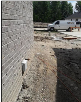
Clear pathway from meter location to street.
